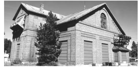
1909 Milwaukee Railroad electric substation in South Cle Elum Railyard. (Photo courtesy of National Trust)
