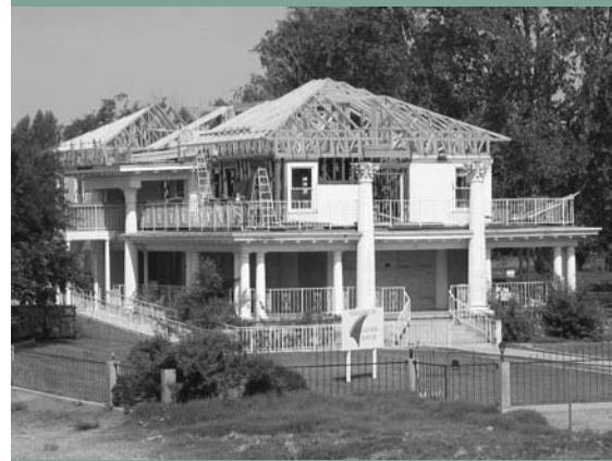
The 1908 Moore House in Pasco is now being restored following significant fire damage in 2001. (Photo by Ange Mills)
