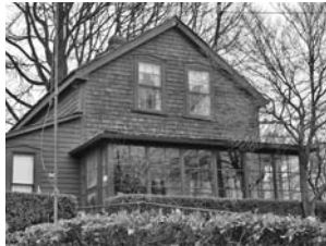
Daughters of the Pioneers of Washington Whatcom Chapter 5, Bellingham —$1,800 to install cedar shakes on the lean-to roof of the Pickett House Museum
