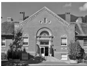
The Cutter Theatre, Metaline Falls —$2,000 to repair concrete bearing walls in the basement and repaint the front parapet of the Cutter Theatre
