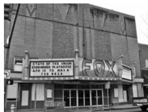
City of Centralia, Centralia —$2,000 to restore the corner storefront of the Fox Theatre
