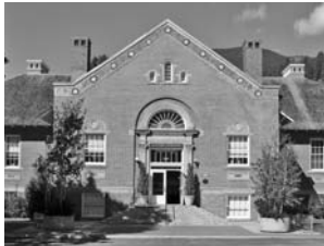
The Cutter Theatre, Metaline Falls —$2,000 to repair concrete bearing walls in the basement and repaint the front parapet of the Cutter Theatre
