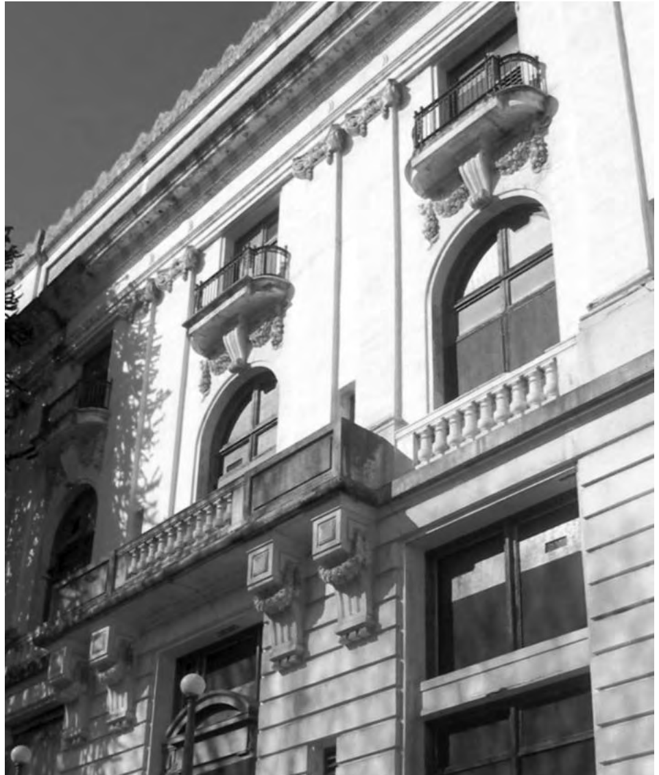
Tacoma's historic Elk's Lodge is slated for major renovation. Photo by Gerry Sperry.
