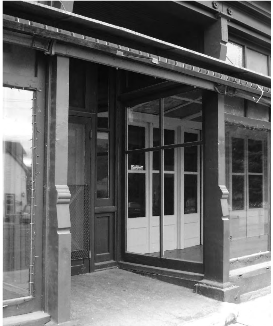
Detail of the NWIC Building doorway showing an interesting cast iron structural storefront framing system that replaced the building's original arched windows (see historic image at left). Photo courtesy of Kevin Kane, SHKS Architects.
