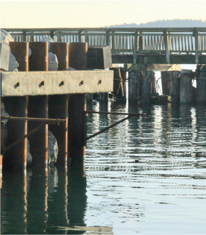
Opposite: Thick-walled steel piles were driven into place by Orion Marine during the fall and winter of 2022-2023, replicating the crib design of the original protective jetty for Point Hudson.
