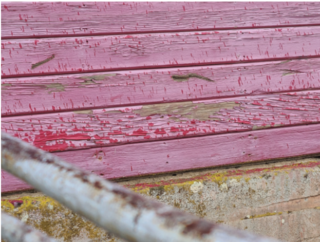
Krause Barn before (left) and after (below). The exterior of Krause Barn was carefully cleaned and repainted, following NPS guidelines.
