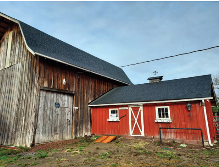
Hull Barn before (above left) and after (above right). To address their leaking metal roof, Hull Farm used grant funds to support the reroofing of the barn with asphalt black three-tab shingles.
