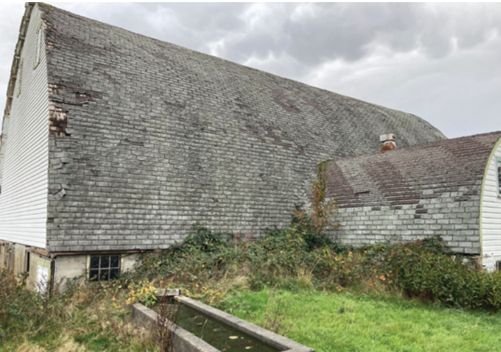
Vekved Barn before (left) and after (above). The existing cedar shake and composite roofing of Vekved Barn were removed and replaced with new composite shingles in accordance with DAHP's standards for roof replacement on heritage barns.
