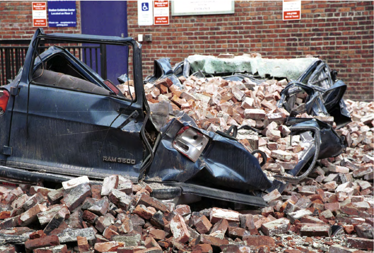
Above: A collapsed URM after the Nisqually earthquake, a moderate event.
