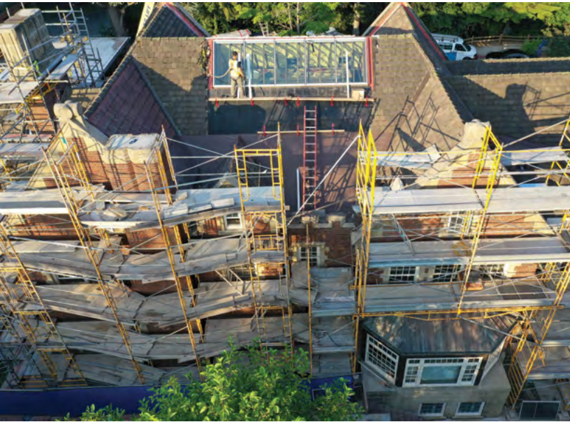
Left: Glass is installed in the building’s new skylight atrium, while scaffolding enables masonry restoration and other projects around the exterior.
