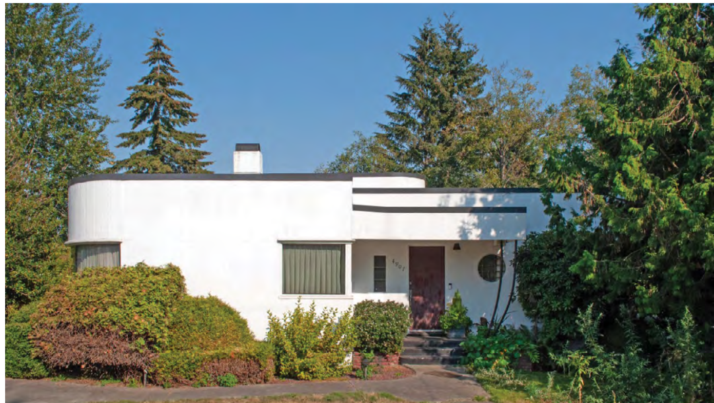
Above: The front of the House of Tomorrow in rural Pierce County. Photo courtesy of Richaven Architecture & Preservation.
