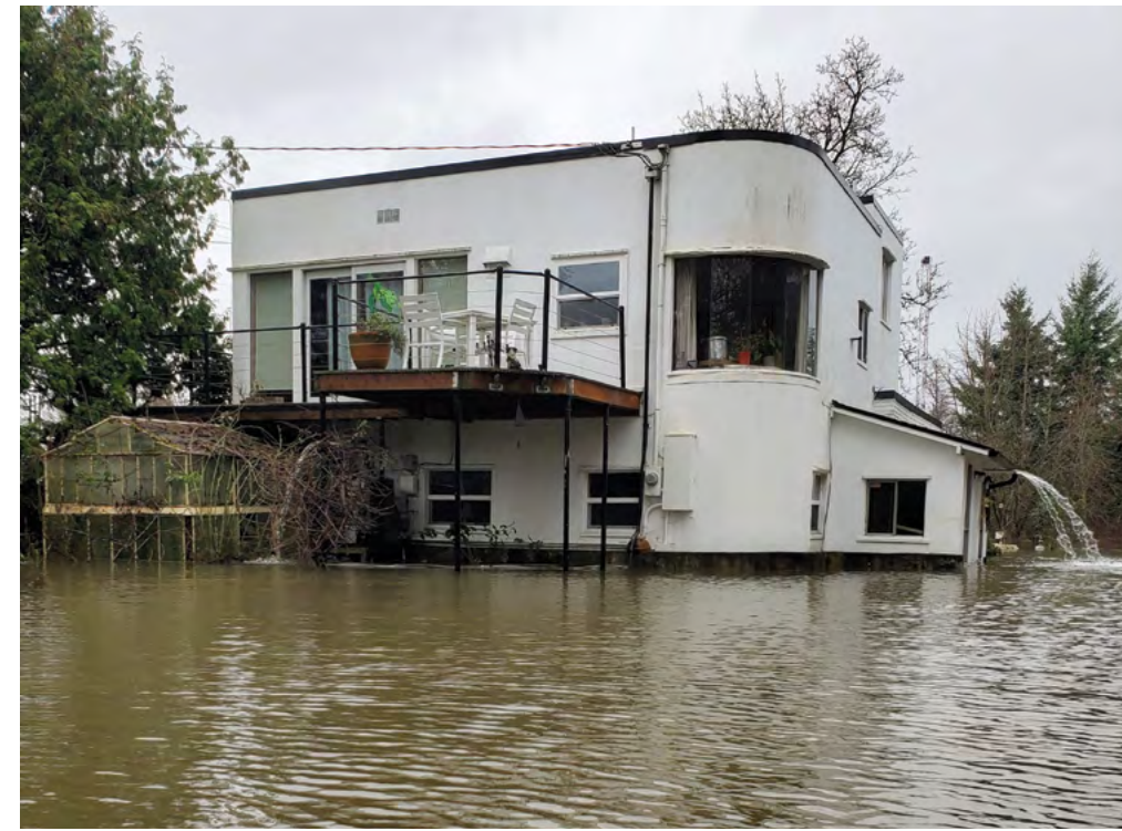
Left: An example of one of the (many) flood events the House of Tomorrow encountered. Photo courtesy of Pierce County.
