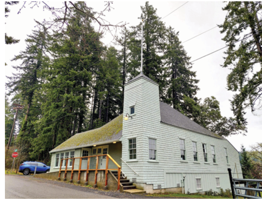
Left: The Key Peninsula Historical Society replaced doors and windows on the historic Vaughn Library Hall thanks to Section 106 mitigation funding, allocated through the Valerie Sivinski Fund. Photo courtesy of the Key Peninsula Historical Society.
