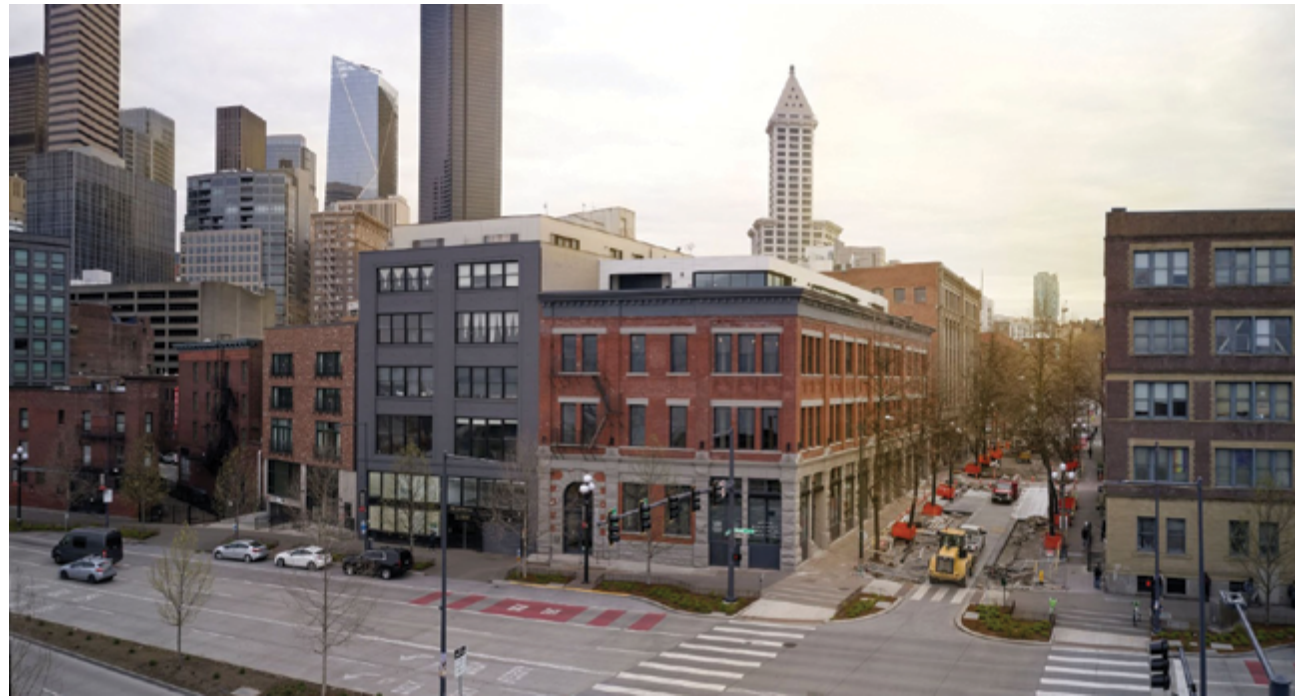
Above: The Washington Park Building in Seattle's Pioneer Square neighborhood recently underwent an extensive building renovation, made possible in part thanks to Section 106 mitigation funding, allocated through the Seattle Historic Waterfronts Grant Program. The project even won Historic Seattle's 2024 Best Preservation Project Award. Photo courtesy of BuildingWork.
