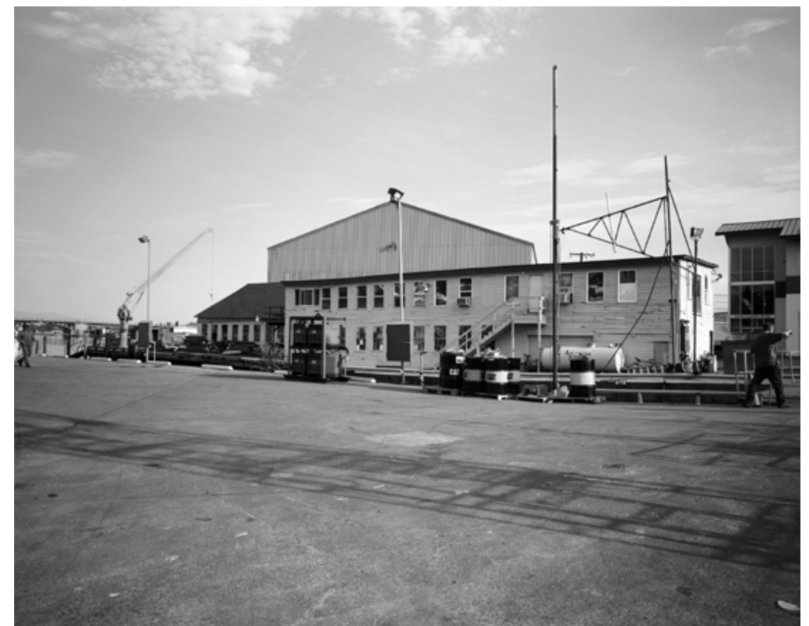
Right: The original Olson & Sunde shop buildings, looking west. Photo courtesy of Abby Inpanbutr.
