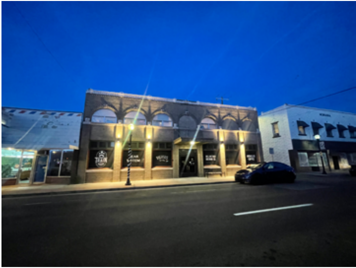
Below: New outdoor sconces illuminate the historic United Building in the Hillyard district.
