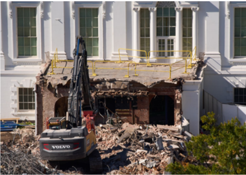
Above: The demolition of the White House's East Wing in Washington, D.C., in October. Photo courtesy of ABC News.
